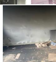
Kitchen Fire Door Removed Closer – Smoke Damage
